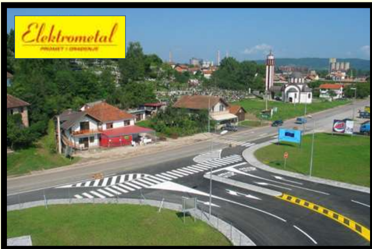
Border Crossing Gradina Jasenovac, B&H
